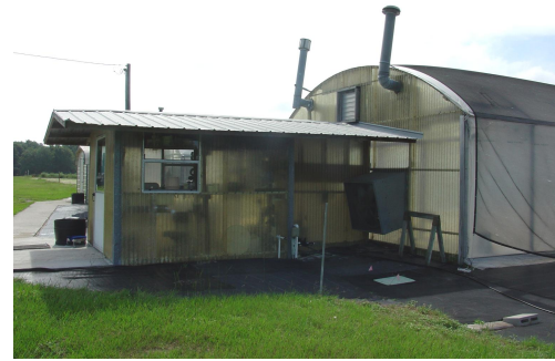
Fig 1. Greenhouse air-lock entrance.
